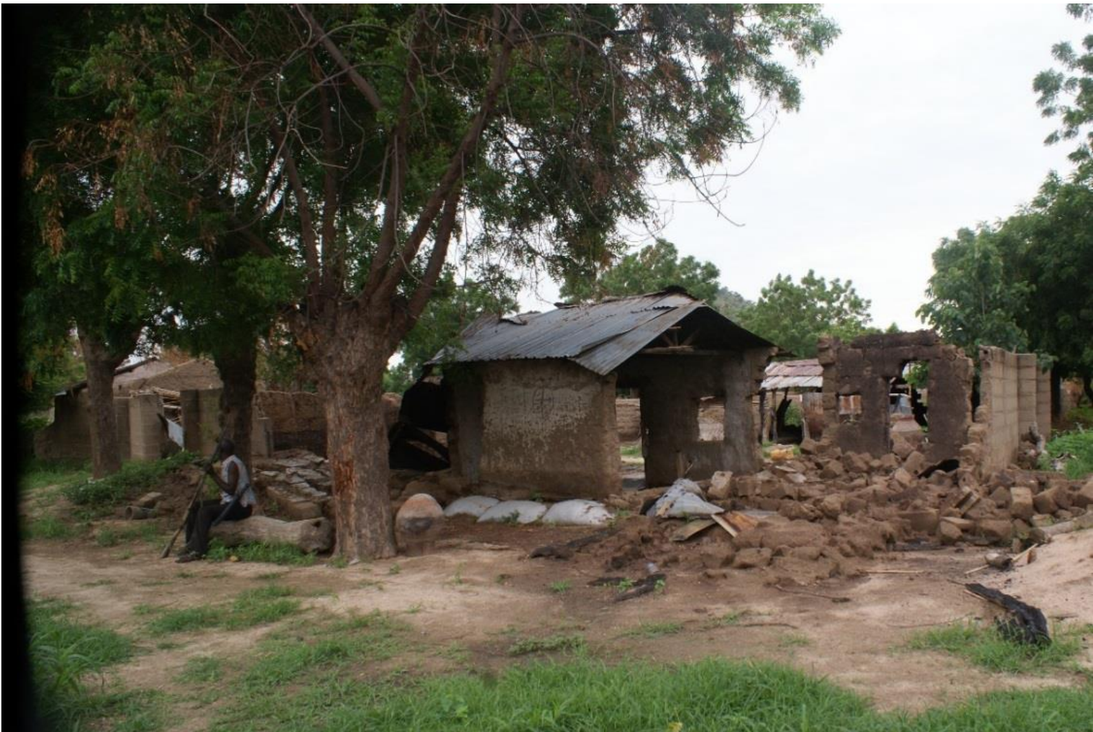
Houses destroyed after a Boko Haram attack in a village in Gwoza LGA. © Private
